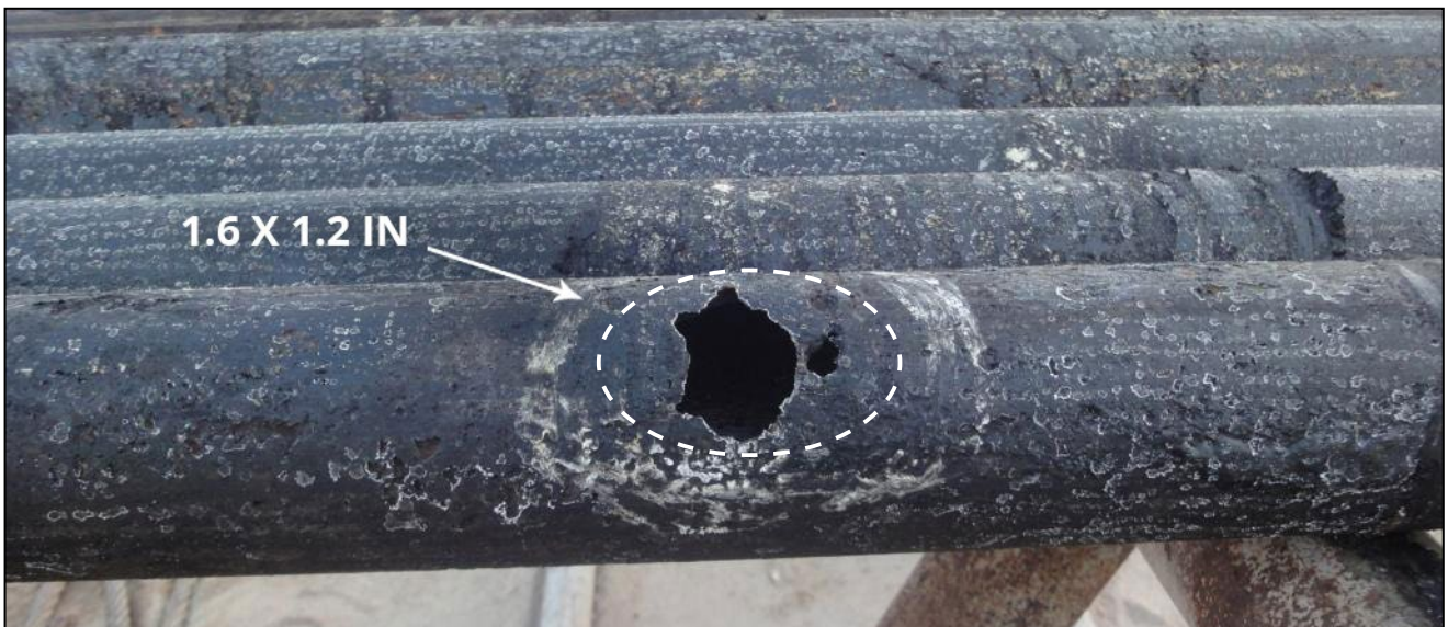
Fig. 1b. Corrosion hole found in the long string at X,907 ft after retrieval
